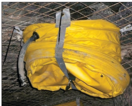
J-CRIB bag attached to wire mesh.
