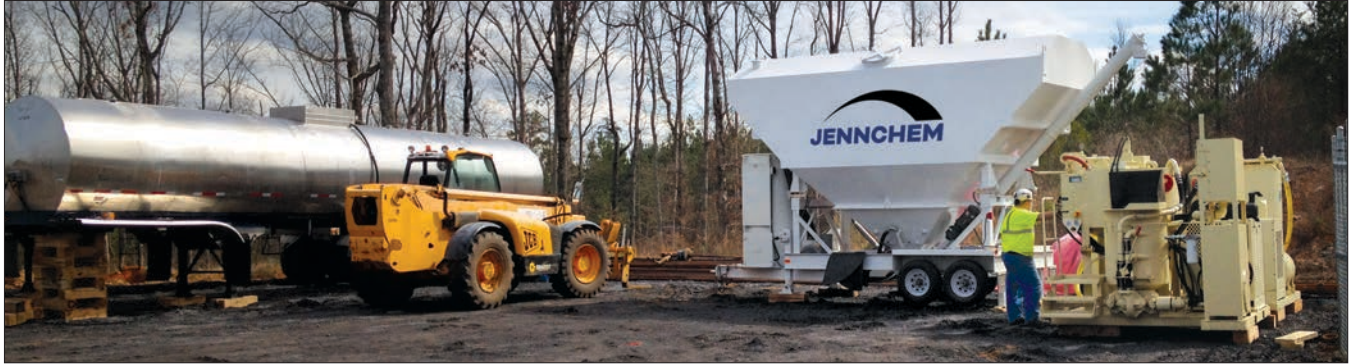
Liquid accelerator tanker, cement hopper, diesel powered mixer & pump system.
