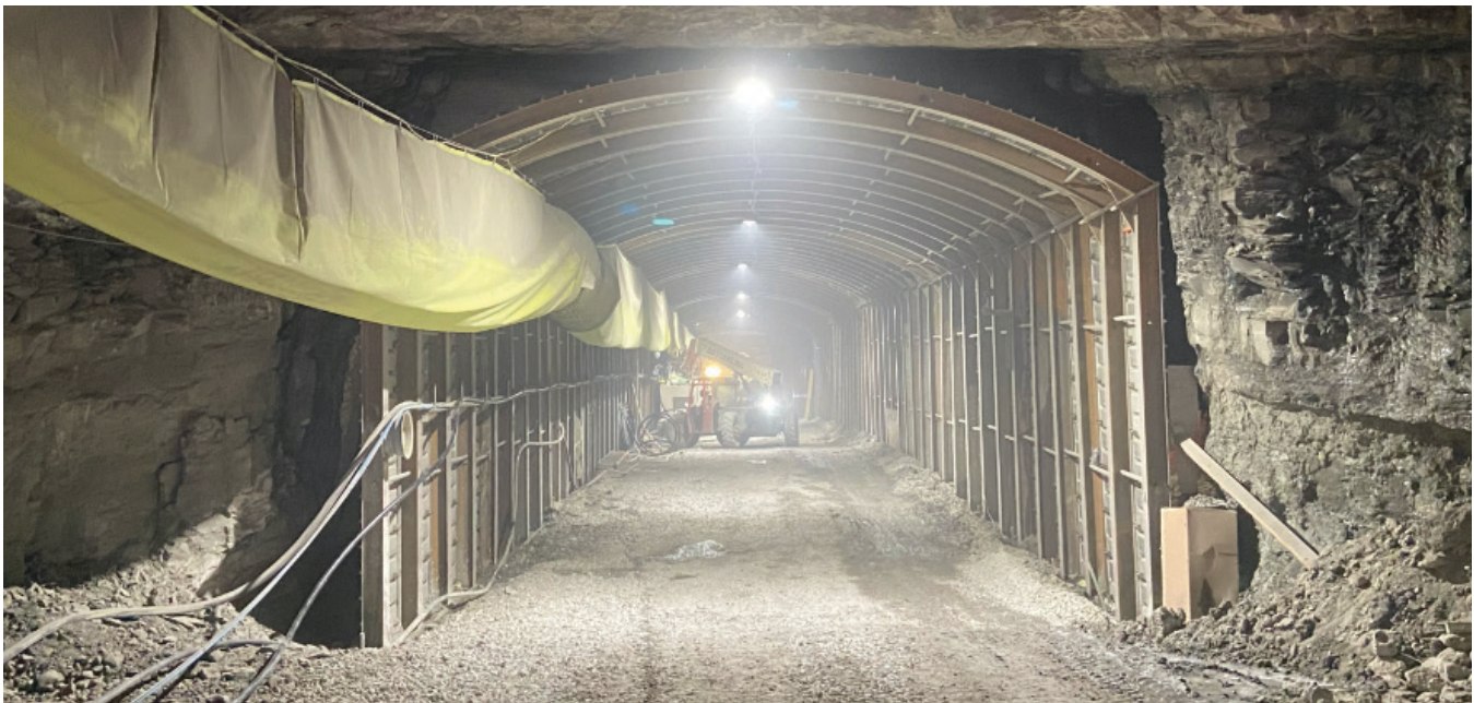
J-SEAL® is a specialized foaming cement which can be used for backfilling behind steel sets or other general backfilling applications in coal or hard rock mining.
