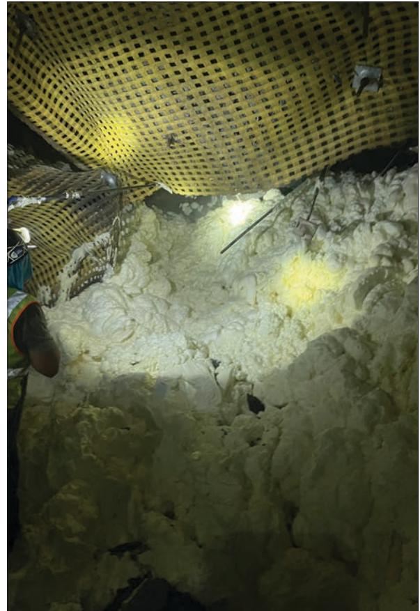
Ultra-X Foam is a two-component grout that is intended for, strata consolidation, coal face reinforcement, and large or small cavity filling.
